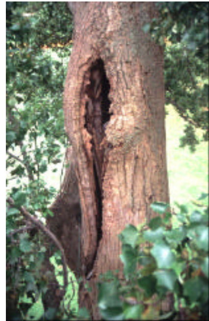
Figure 4 A large cavity at 32 feet in the main trunk, on the north side. There are steel bolts and concrete filler in this cavity.
